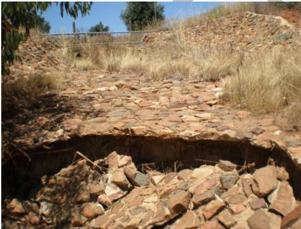
Figure 11 Undermining of Inlet Channel
