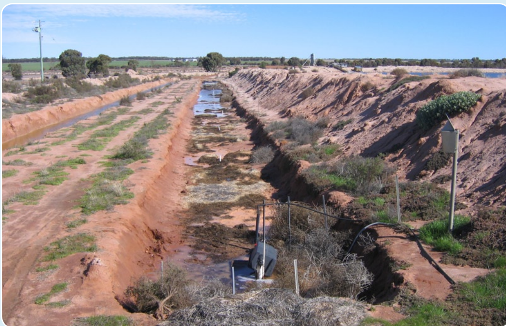
Figure 3 A composting bed in a pit constructed at the end of a drain near Beacon
