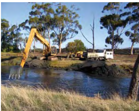
Long-reach excavator removing sediment from the pool. (Photo courtesy Michael Allen)
