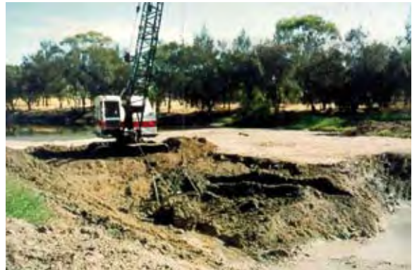
A dragline removing sediment from Beverley Town Pool in 1993 (Photo courtesy Fred Bremner)
