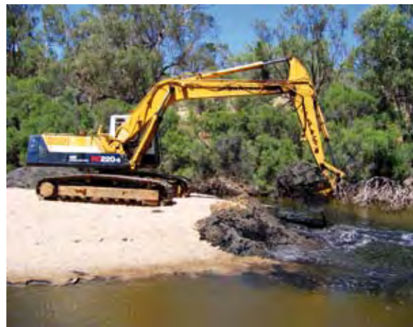
Sediment extraction at Long Pool, Feb 2005 (Photo courtesy Bernard Kelly)
