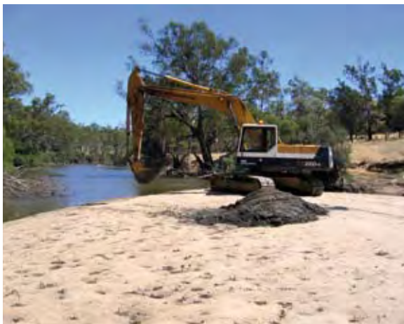
Sediment extraction at Long Pool, Feb 2005 (Photo courtesy Bernard Kelly)
