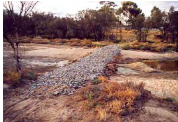
Riffle constructed upstream of Beverley Town Pool to trap sediment (Photo courtesy Bernard Kelly)
