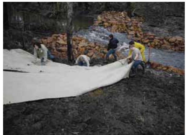
Figure 4. Placing geotextile fabric on the restoration site. (Photo Jesse Steele)
