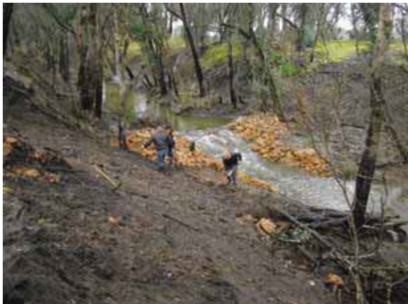
Figure 3. Construction of the riffle. (Photo Jesse Steele)
