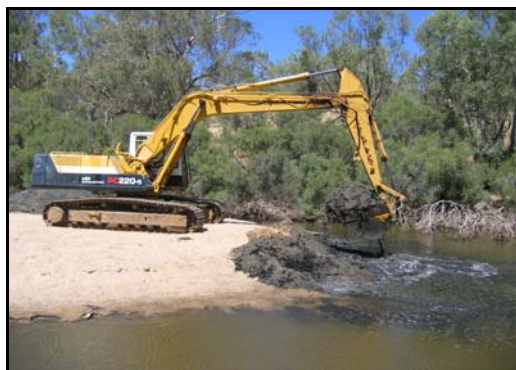
Excavation of coarse sediment from Long Pool February 2005 (Photos courtesy of B. Kelly)
